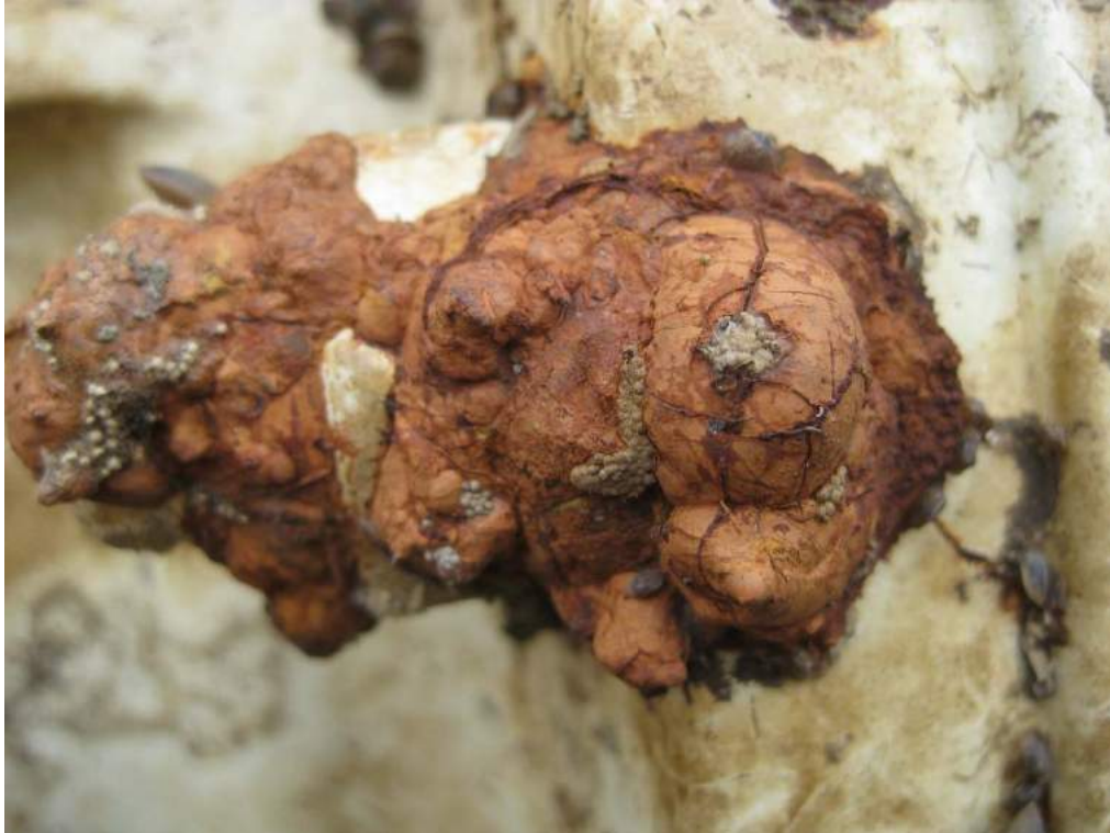
Figure 3: Pump No. 1 Bolt Corrosion Detail
