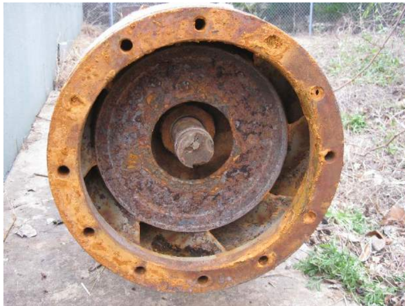
Figure 1: Flange Separation at Stage 2 in Pump No. 1
