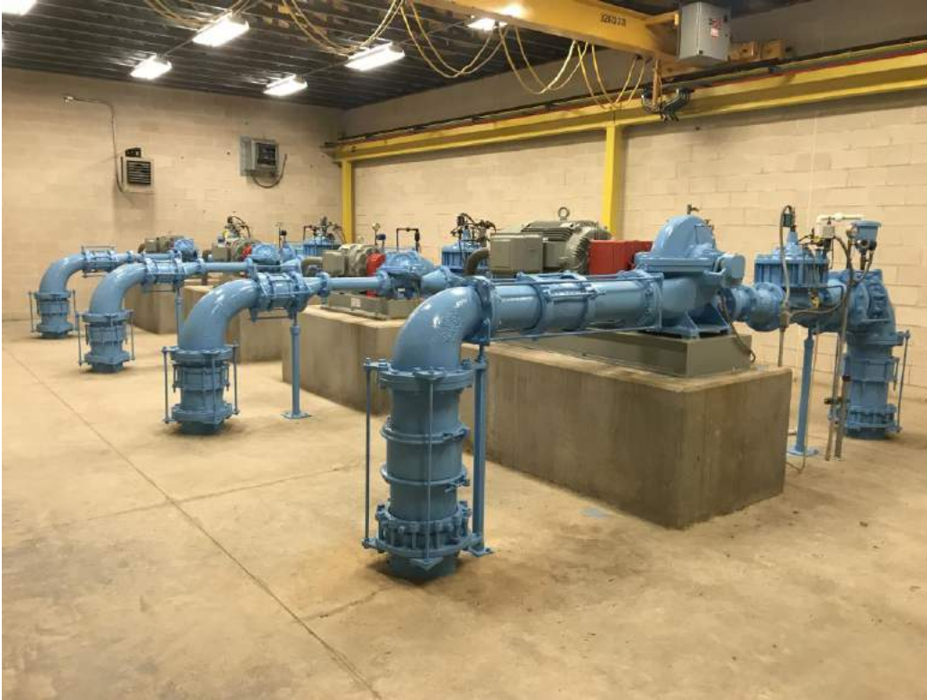
West Bee Cave Pump Station
