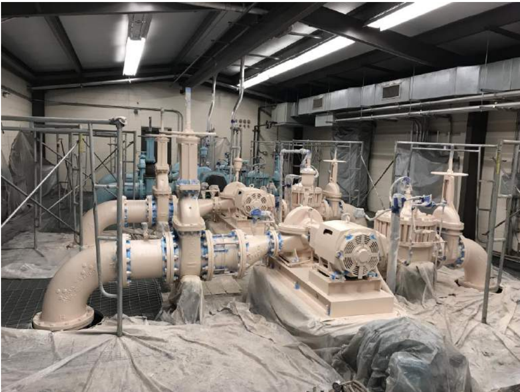
County Line Pump Station
