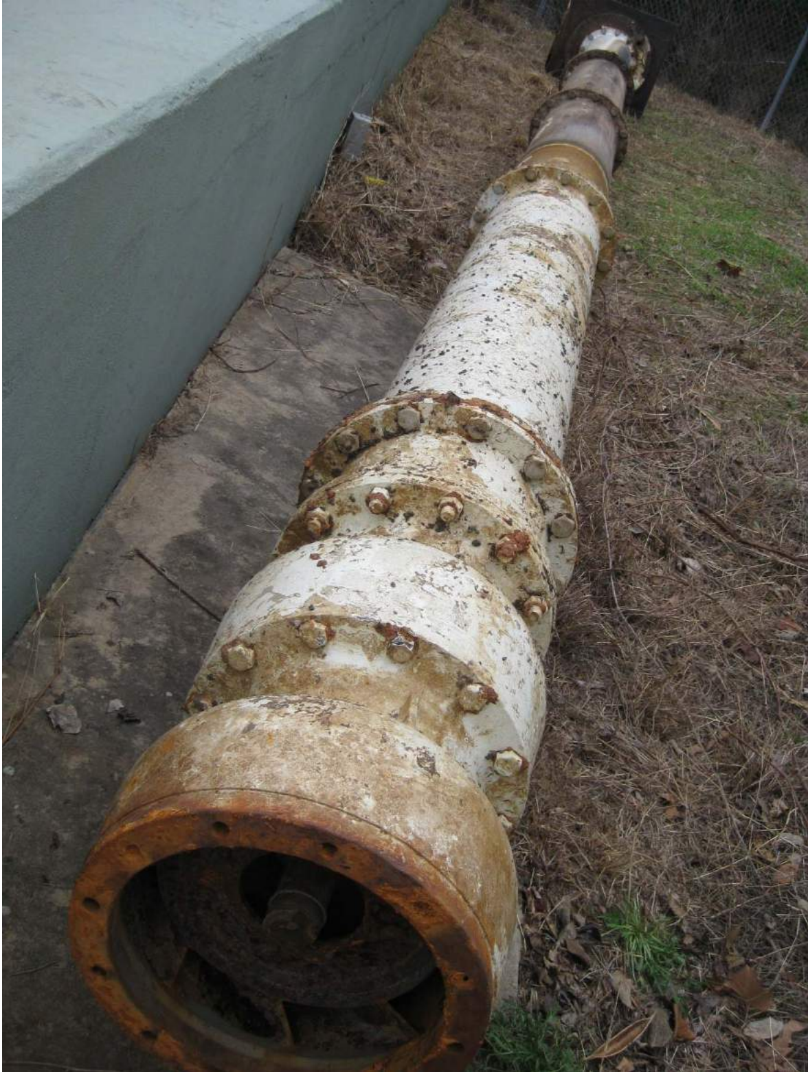
Figure 2: Pump No. 1 Remaining Pump Assembly
