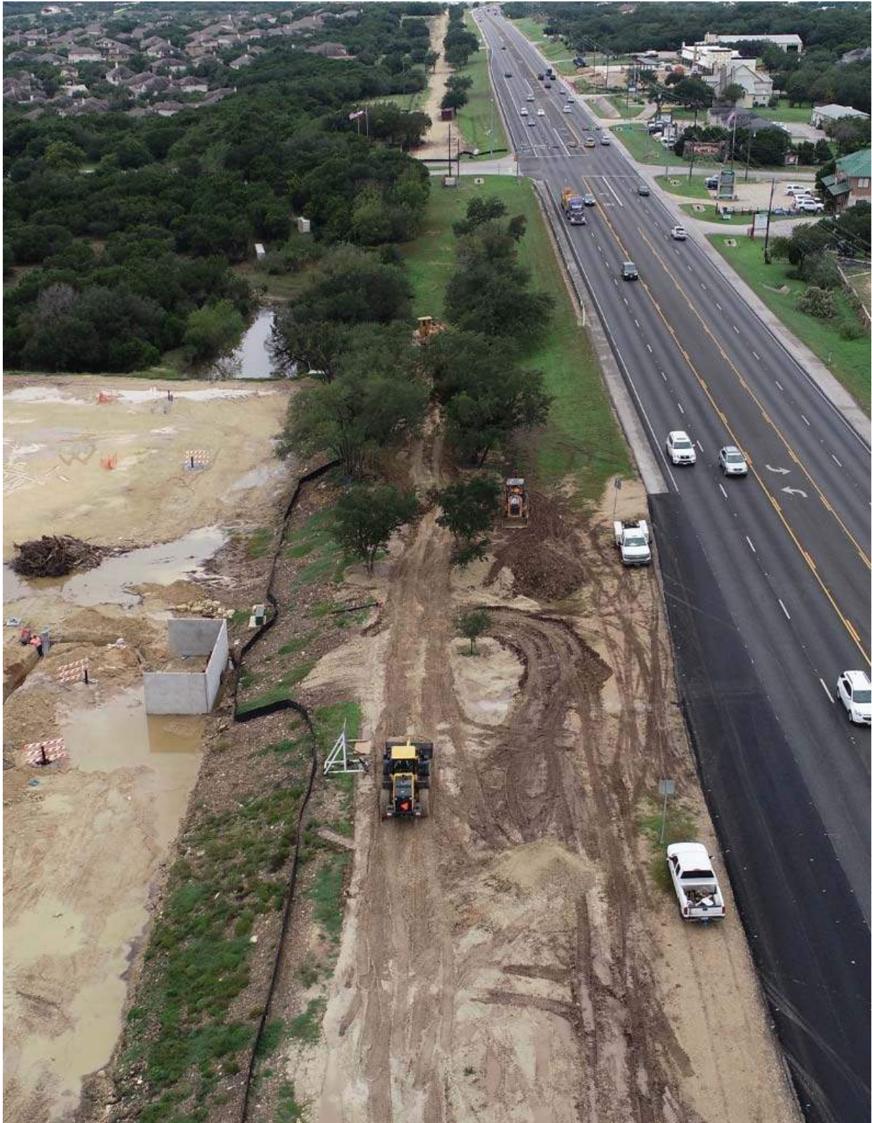
1340 Transmission Main Trenching
