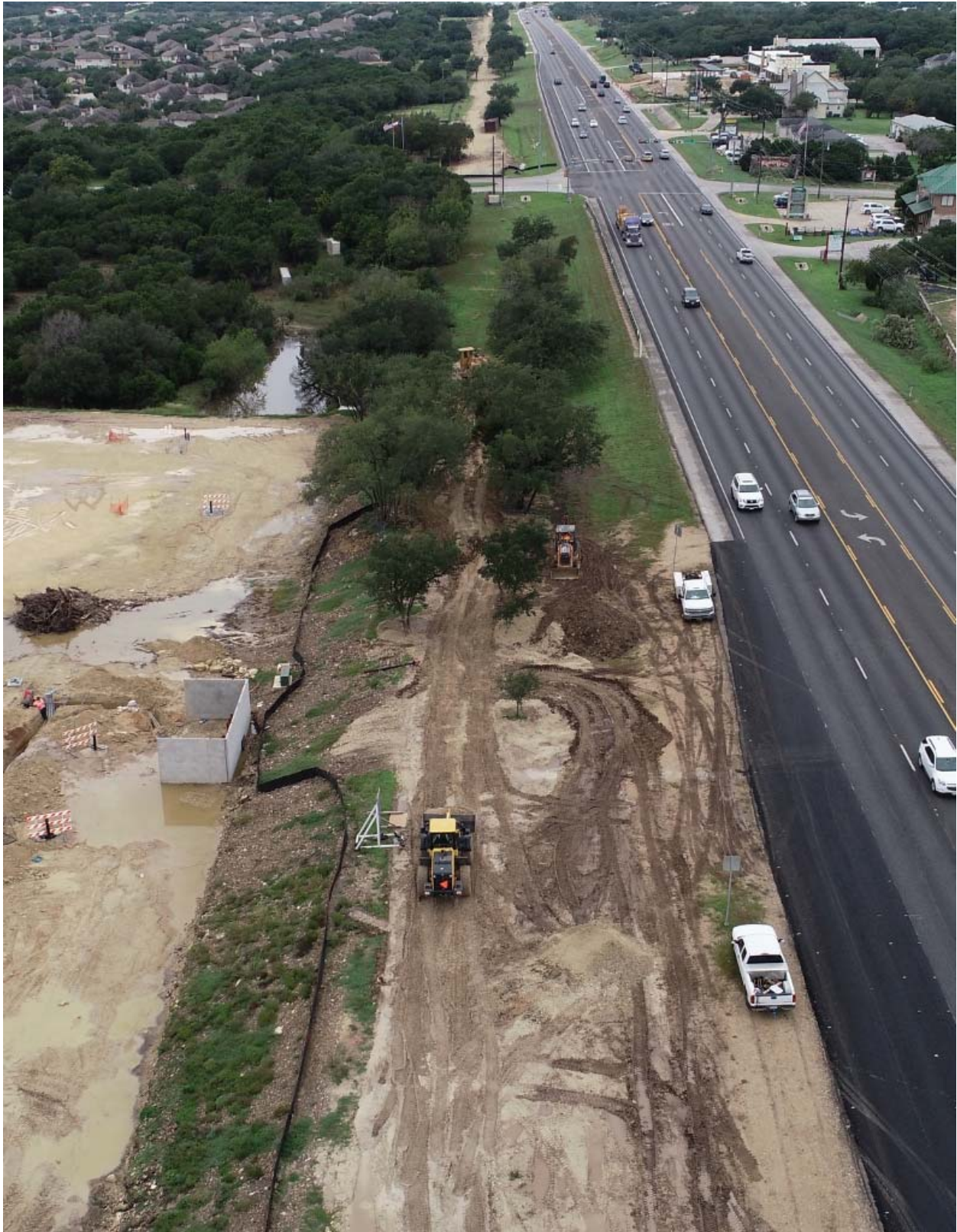
1340 Transmission Main Trenching
