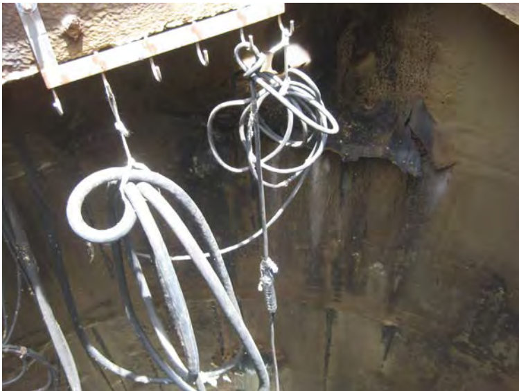
Figure 2: Failure of wet well coating
