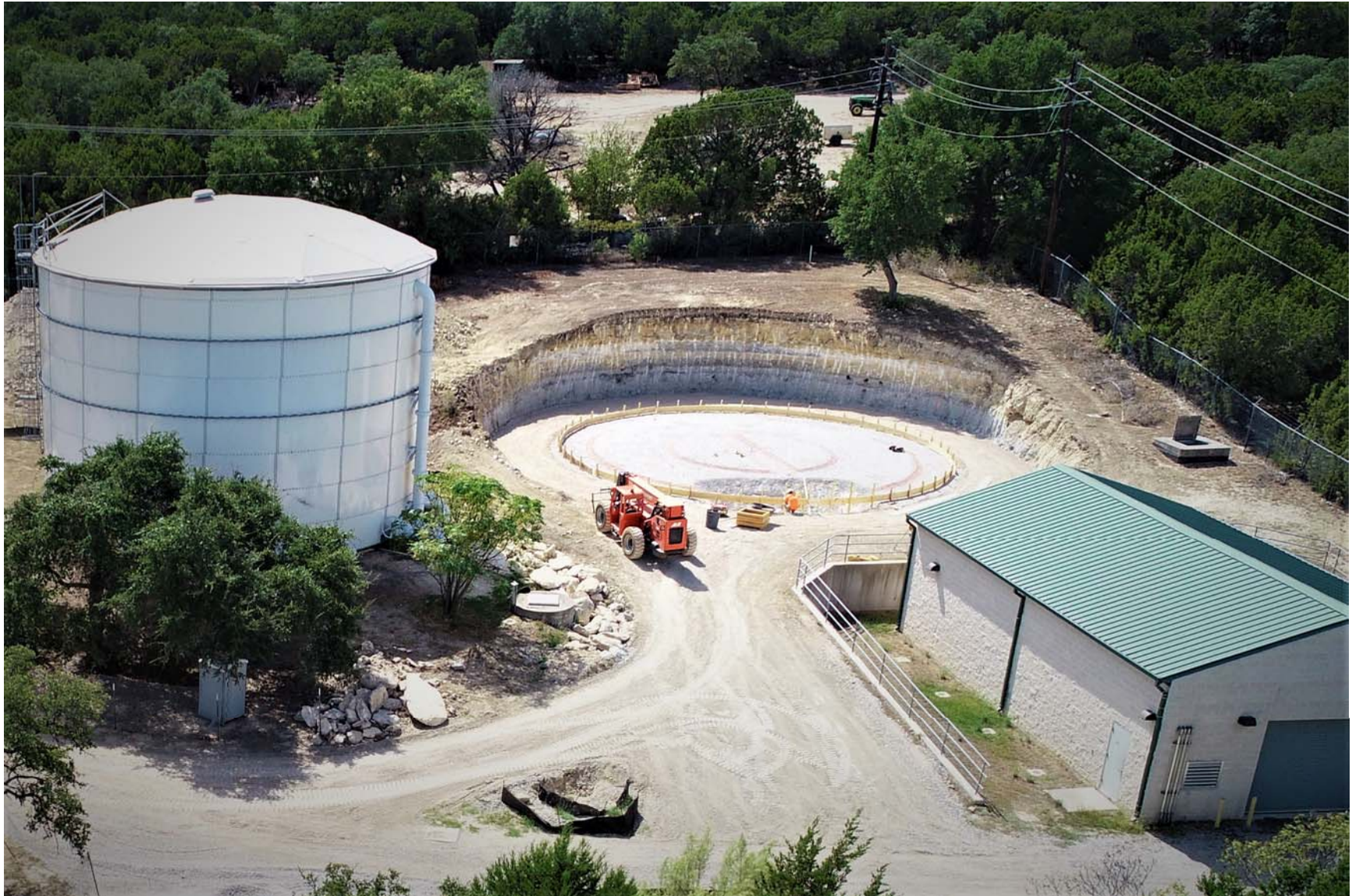
Bee Cave Pump Station GST 2 Site
