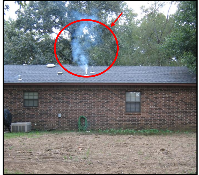
Smoke may exit from the vent pipe on top of each residence during smoke testing.
